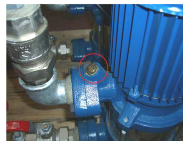
Fig. 8: mounting transducer to venting air hole on the delivery pump
